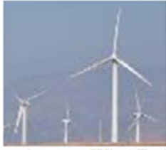
Atrin Development Wind Turbines Co.
